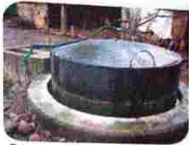
Fig. 1.10 Biogas digester, Type Kubah Tetap.
